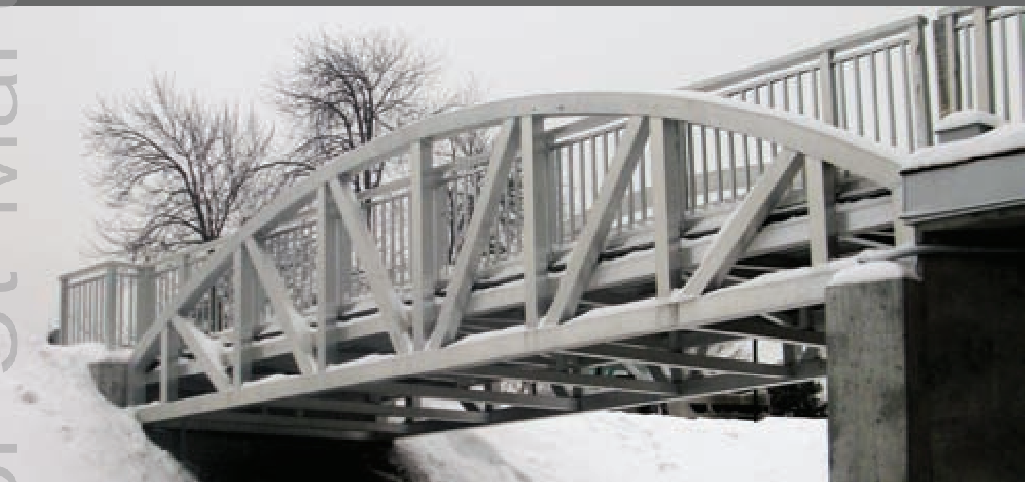
Aluminum pedestrian bridge October 2008 Laval, QC
