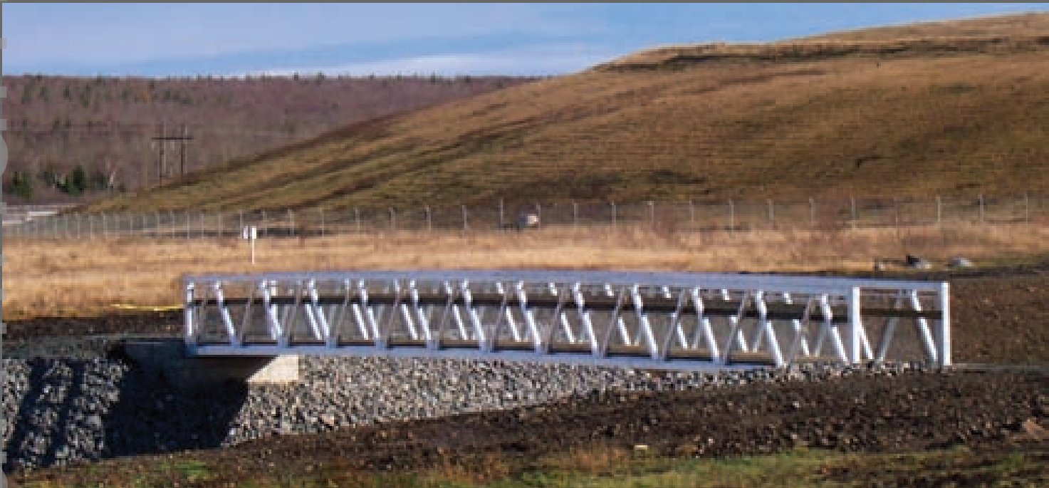
ATV aluminum bridge November Sydney, N-S 2006
